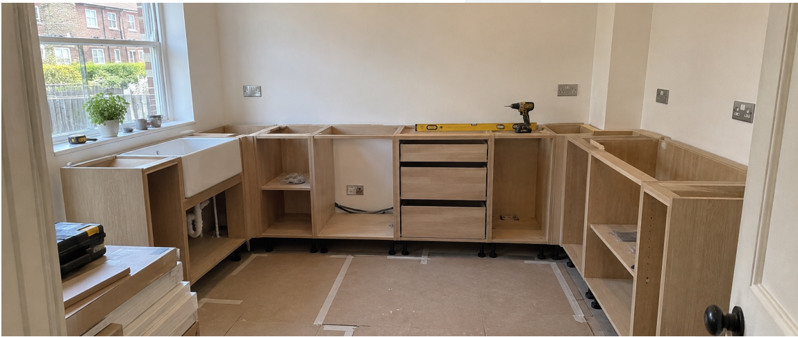
01 Base cabinets positioned and levelled.
