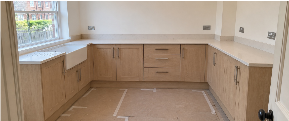
02 Worktop and doors fitted; final checks to follow.
